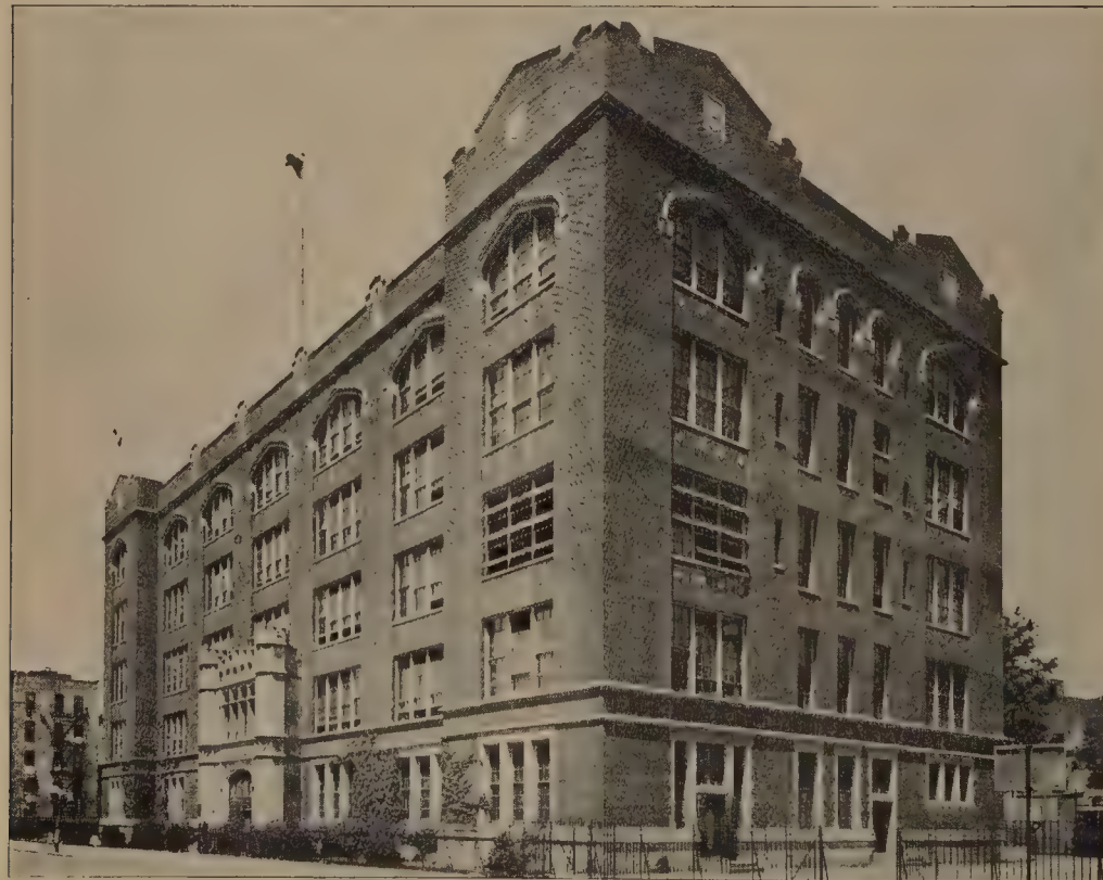
576 W. H. Gompert, architect; photograph by courtesy of the Board of Education, New York
